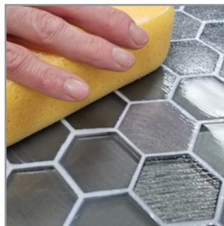
Then, using a slightly dampened sponge (not wet), gently wipe excess material from the surface using light and delicate diagonal passes. Change water and rinse the sponge frequently. Keeping the water and sponge clean will achieve better joint color uniformity.
