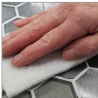
Allow grout to harden for about 20 to 30 minutes. Using a slightly dampened white scrubbing pad, loosen up all excess grout over the tile with a circular motion. Do not add water before everything is well loosened up.
