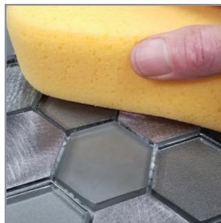
Slightly moisten tile surface with a damp sponge just before application to help with spreading the grout.
