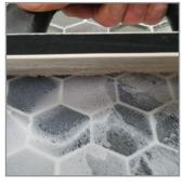
With a firm to medium sharp-edged rubber float, force grout diagonally into the joint at a 45° angle, ensuring that the grout is wellcompacted, free of voids and pin holes, and filled flush with the tile or stone edge.
